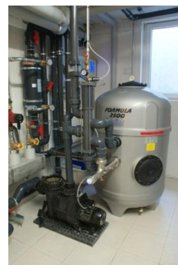
UV sterilisation of swimming pool water
