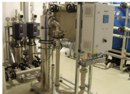
UV treatment for TOC reduction
